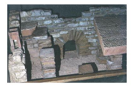
A hypocaust was underneath the floor of a room. It was the Roman central heating system.
